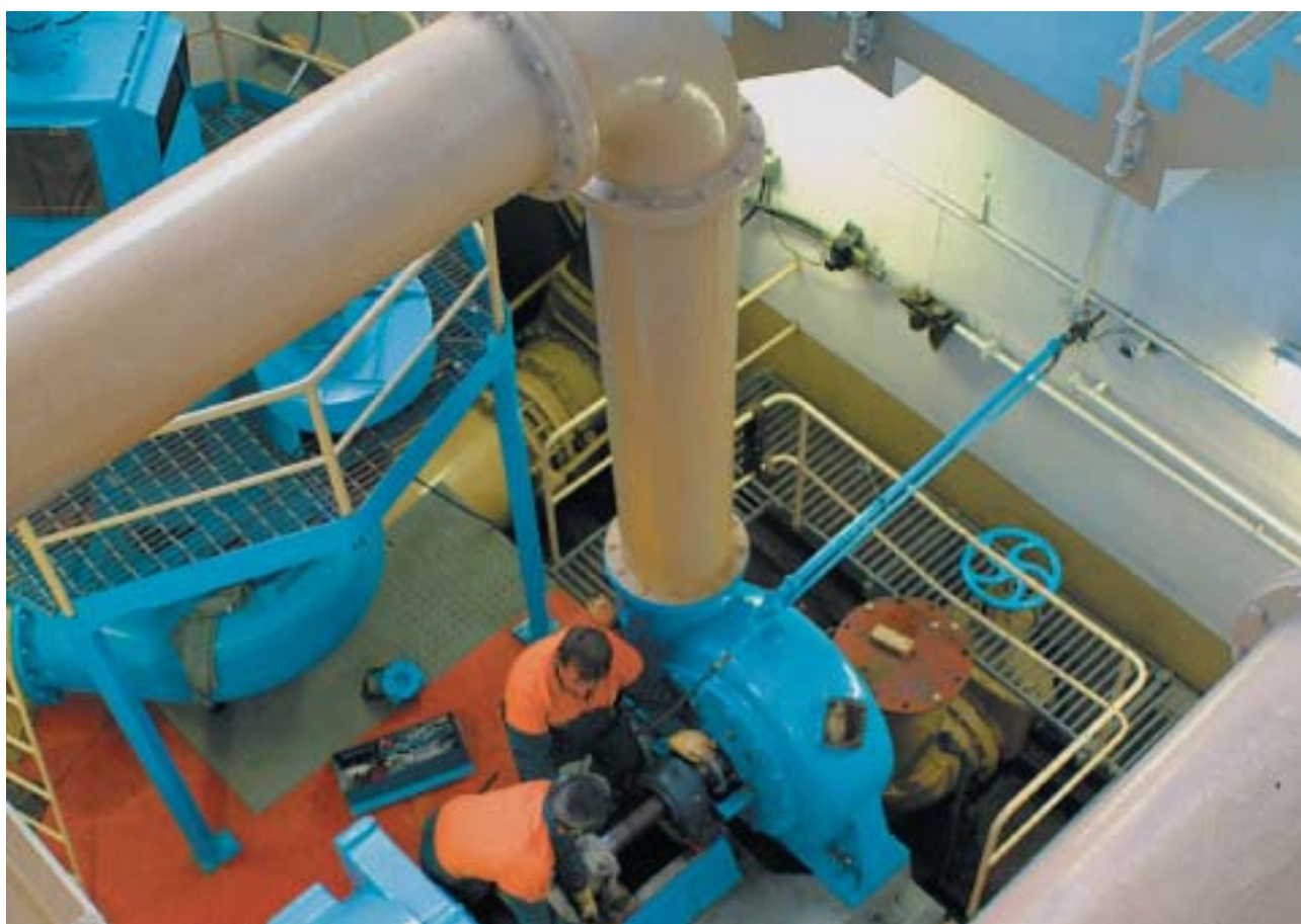
City Care staff conducting pump maintenance for the City Council.
