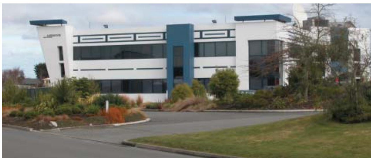
One of the Airways Corporation buildings in the Canterbury Technology Park.
