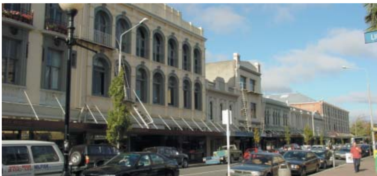
Historic buildings in High Street where heritage precinct work was completed during the year.
